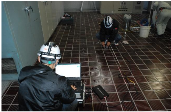
2mスラブ下空洞探査
